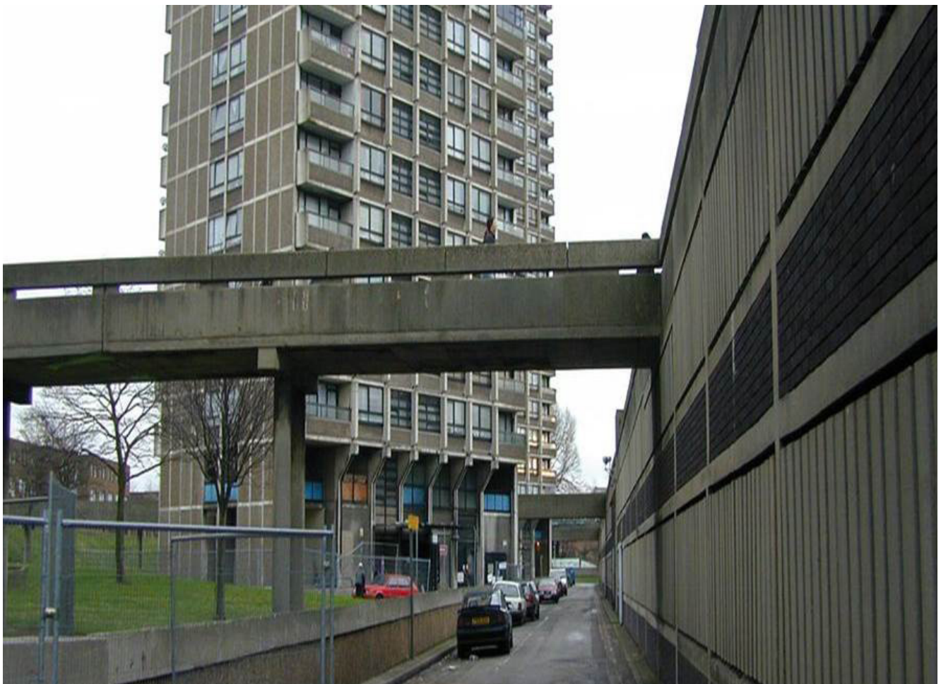
CROSSWAYS ESTATE BEFORE EXTENSIVE REFURBISHMENT, TOWER HAMLETS
