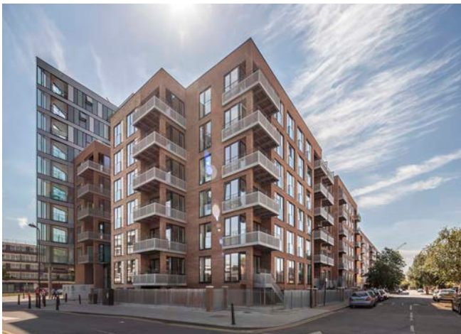
HAGGERSTON AND KINGSLAND ESTATE, HACKNEY
