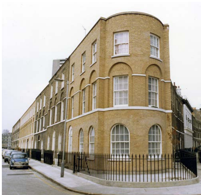
WOODBIDGE ESTATE, ISLINGTON – FULLY INTEGRATED WITH ITS SURROUNDINGS
