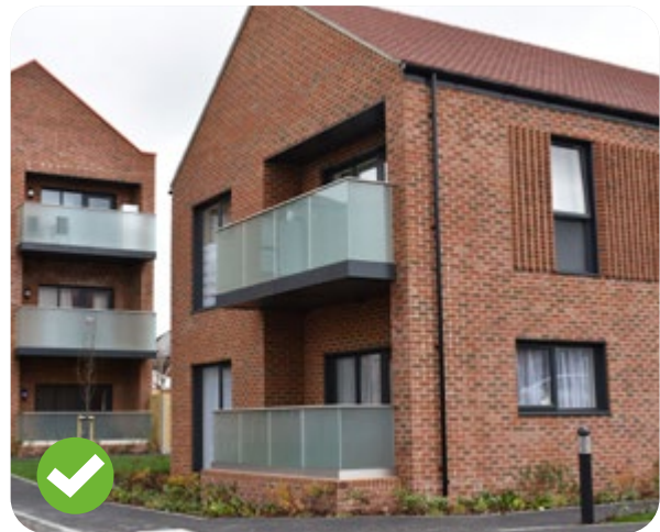
Fig 139 Semi-recessed balconies provide protection from adverse weather while integrating façade's rhythm and articulation (Pankhurst Place)
