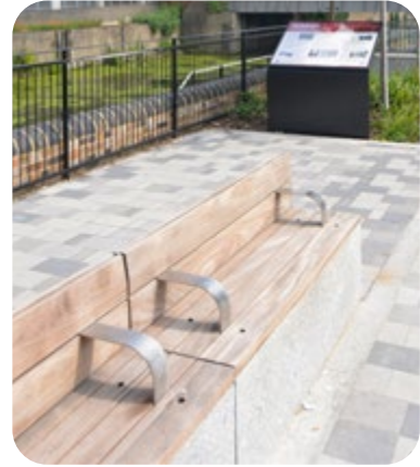
Fig 68 FSC certified hardwood timber seating walls with sections including arms and backrests
