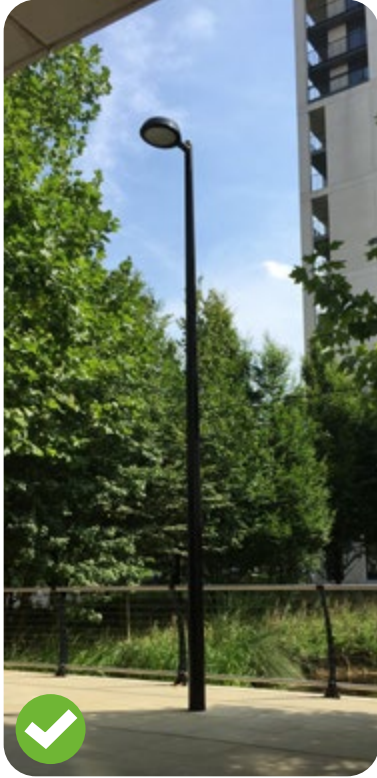
Fig 74 Columns in vehicular areas that are simple, robust, with consistent colours at 5-7m high
