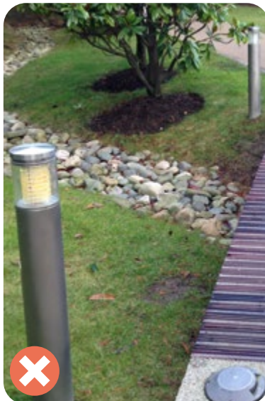
Fig 78 Bollard-style lighting can contribute to clutter and often become maintenance issues
