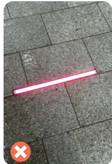
Fig 79 In-ground lighting fittings can become maintenance issues if not specified correctly
