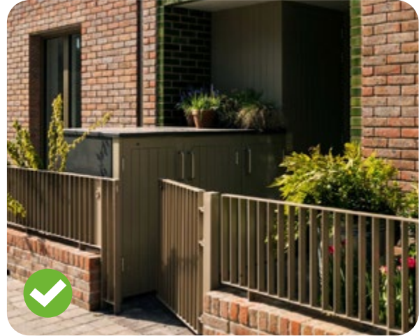
Fig 161 Bike store integrated within the design of the dwelling entrance (Dujardin Mews by Maccreanor Lavington)
