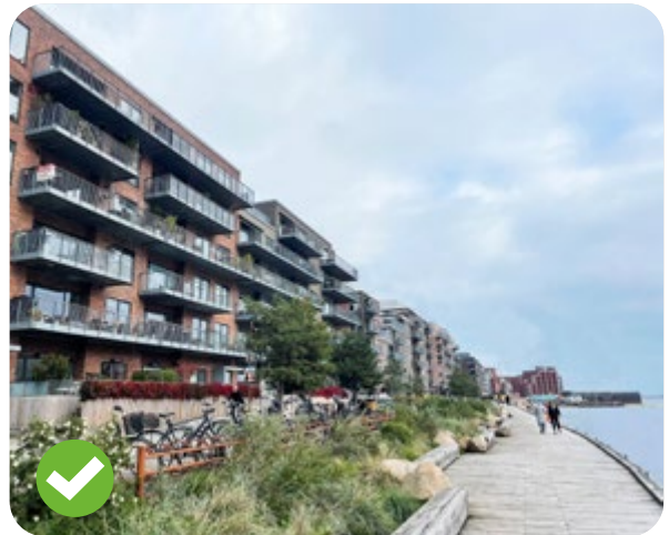
Fig 177 Housing set back from the riverside allowing for a generous public realm for pedestrians and cyclists (Sandkaj by Mikkelsen Arkitekter)
