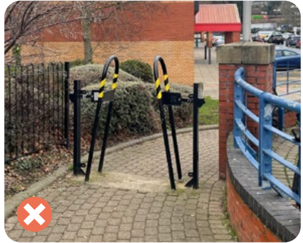
Fig 175 Avoid excessively engineered approaches to riverside access
