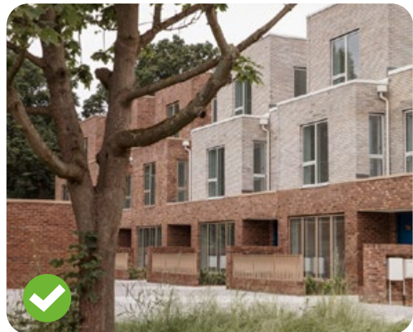
Fig 122 A darker brick is used to reinforce the importance of the ground floor and dwelling entrances (Marston Way by Stitch)
