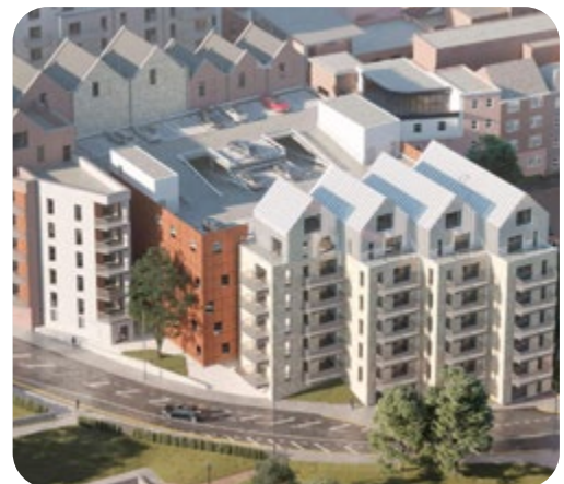
Fig 158 Development with a multi-level car park (The Charter in Gravesend by Leslie Jones Architects)
