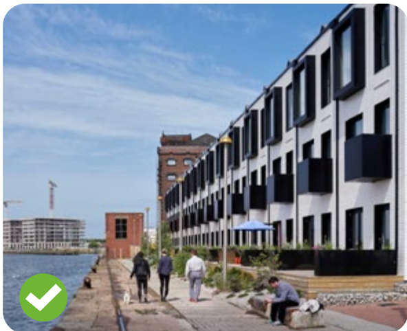
Fig 178 Housing along a riverside promoting walking and cycling (Redbridge Quay by Shedkm)
