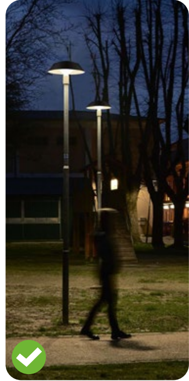
Fig 76 Along pedestrian-only routes, columns drop in height to 3-4m with consistent colours
