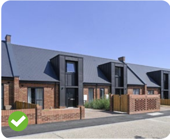
Fig 85 Façade is broken into smaller bays by dormers and door entrances (Constable Road by BPTW)
