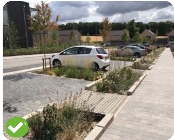
Fig 148 Example of how to integrate sustainable drainage systems (SuDS) such as permeable surfaces and rain gardens to add biodiversity in parking areas
