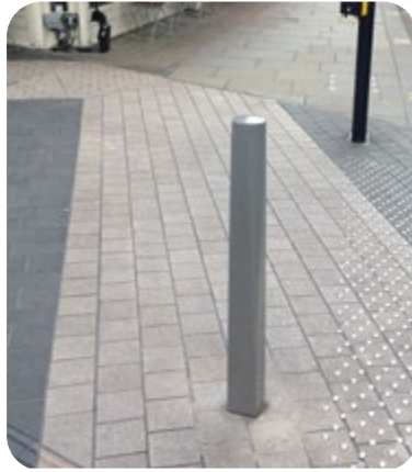
Fig 70 Slim yet robust static bollards in consistent colour palette with demountable option
