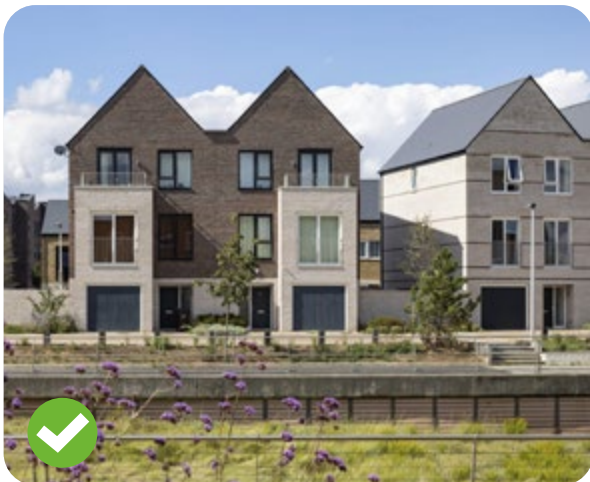
Fig 140 Set-backs in the building façades are opportunities for terraces (Rochester Riverside by BPTW)
