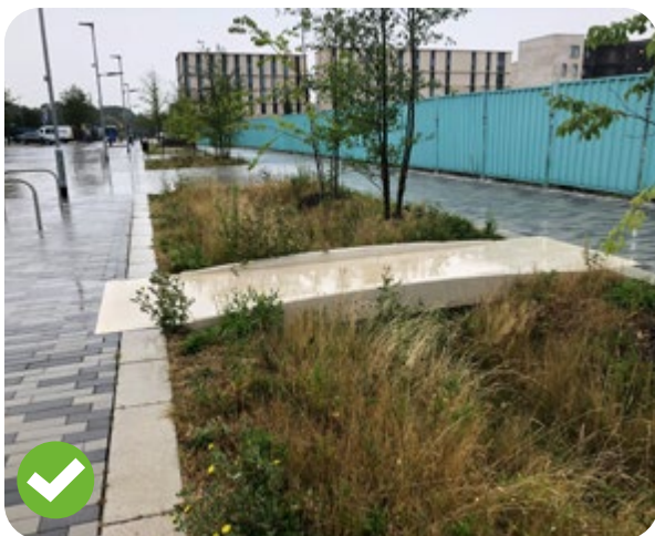
Fig 171 Example of a linear, planted bio-swale contributing to plant diversity
