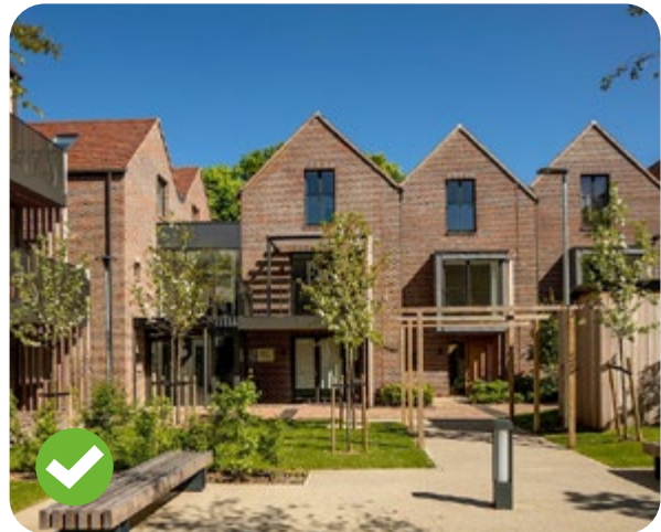
Fig 132 Private balconies facing communal courtyard (Woodside Square by Pollard Thomas Edwards)
