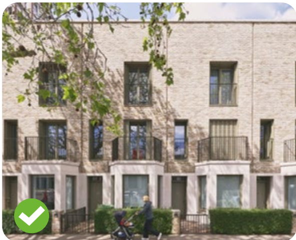
Fig 180 Contemporary townhouses designed to passivhaus principles (South Garden by Maccreanor Lavington)
