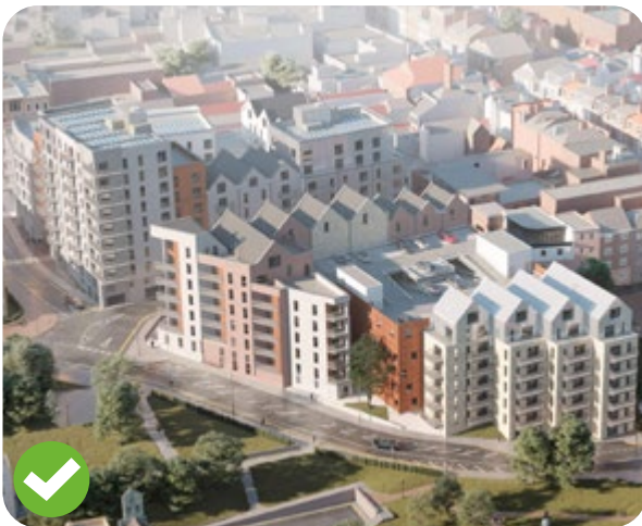
Fig 91 Development with a multi-level car park (The Charter in Gravesend by Leslie Jones Architects)
