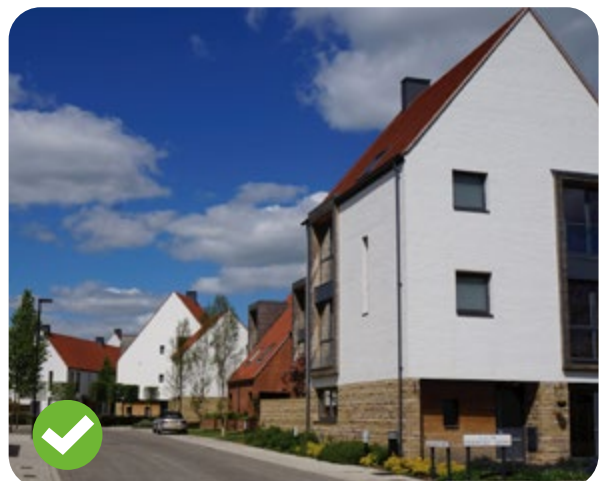
Fig 112 Landscape along the threshold can help soften the transition between dwelling and public realm while enriching the character of the street (Derwenthorpe by Studio Partington)
