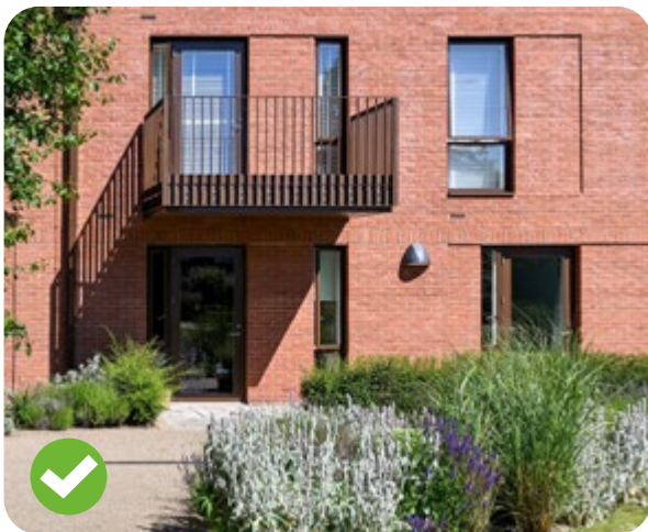
Fig 138 First floor projecting or semi-recessed balconies can provide a canopy over main dwelling entrance (New Lodge Community by PRP)
