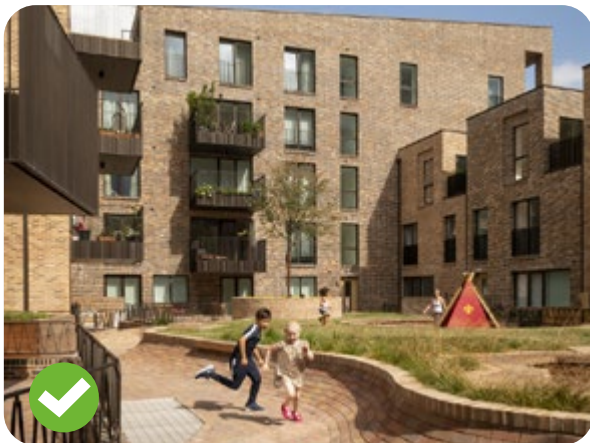
Fig 130 Communal garden within a courtyard building (Branch Place by Karakusevic Carson Architects)
