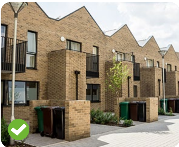
Fig 160 Bin store incorporated within the design of the dwelling entrance (Pump House by Levitt Bernstein)
