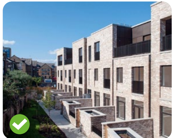
Fig 88 Set-backs and brick recesses can help articulate the elevation of a building (Great Eastern Buildings by Karakusevic Carson Architects)
